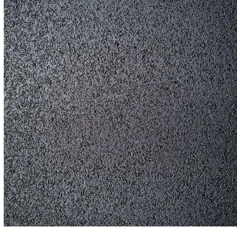
Vehicle areas - Asphalt
