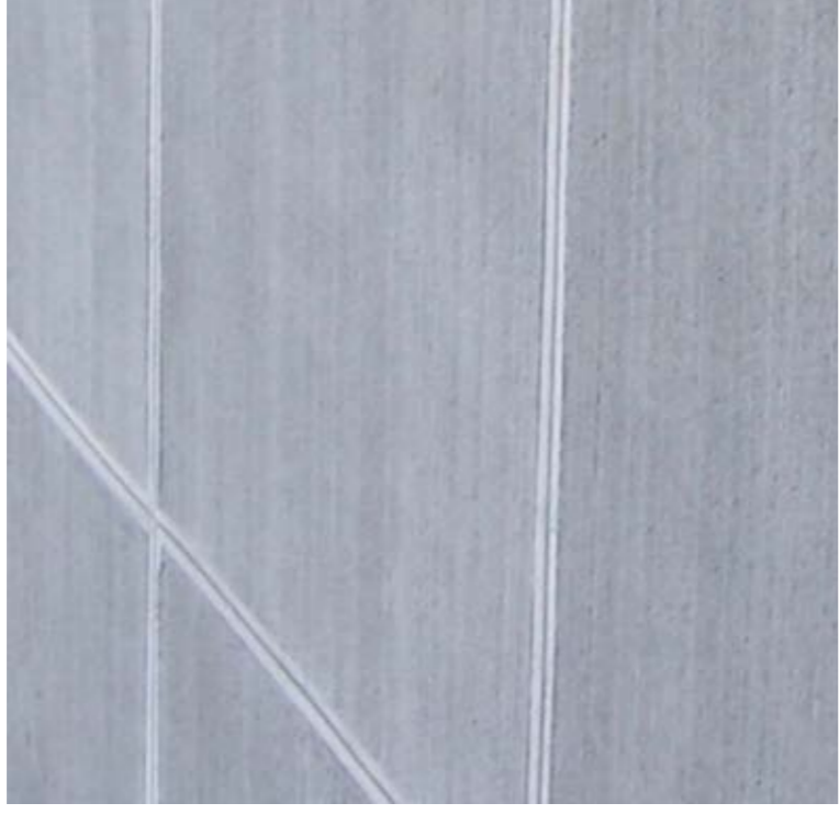
Secondary Path - Broom finished concrete
