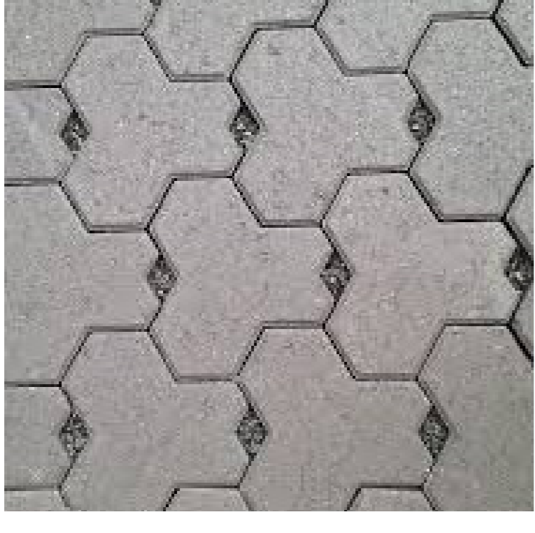
Vehicle areas - Interlocking concrete unit pavers
