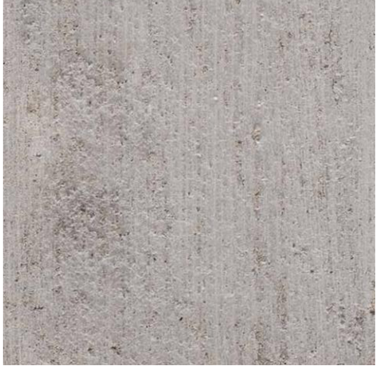
Primary / Secondary Path - Coloured concrete
